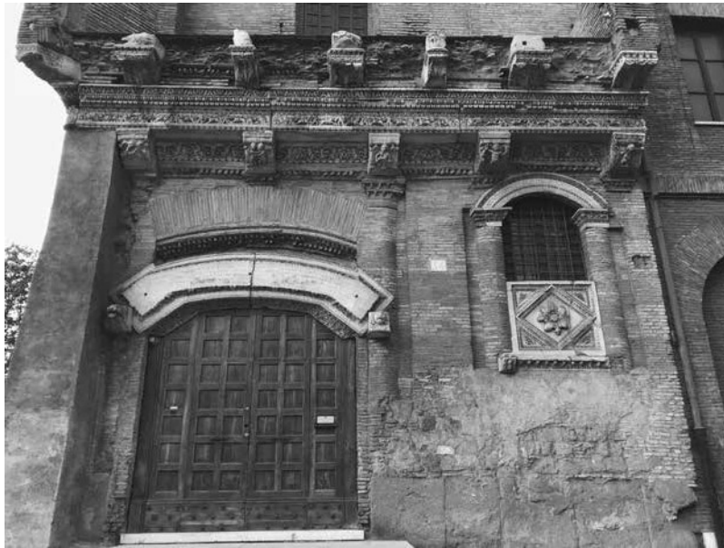
Pieces of Roman marble built into a medieval house. The façade of the tenth-century House of the Crescentii in Rome. Author's photo
